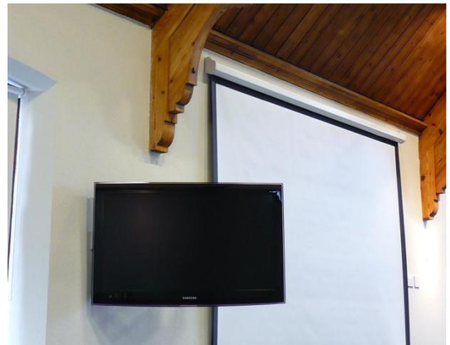
Picture showing one of the wall mounted LCD displays mounted on a Z-bracket for angling to different areas of the congregation depending on room orientation. Via a custom designed four-output PC, every display has the option of showing either the main projection information, working screen or desktop as preferred.
