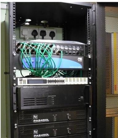
AV Rack containing all amplification, the EV DC-ONE speaker processor and AV connection patch bay utilising Kramer Cat5e cabling and hardware for the highest image quality.
