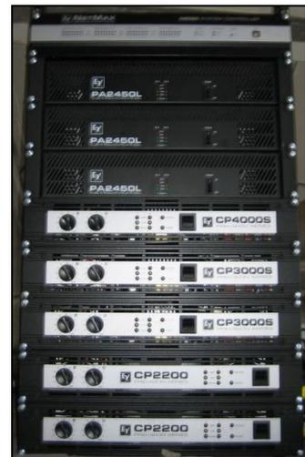
**Amplifier and control rack featuring an EV Netmax control system and front of house speaker amplification**
