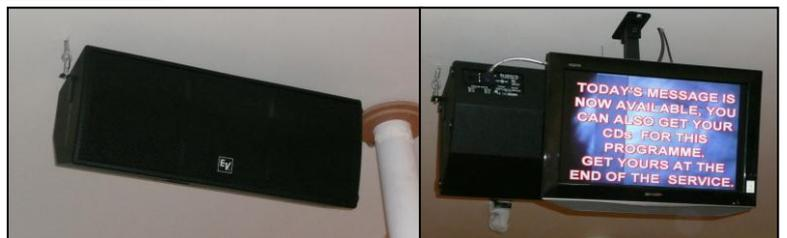
The audio system comprises of ceiling mounted Electrovoice Rx speakers including the Rx212H shown above which is designed for horizontal mounting with a rotatable 3" central compression driver.
