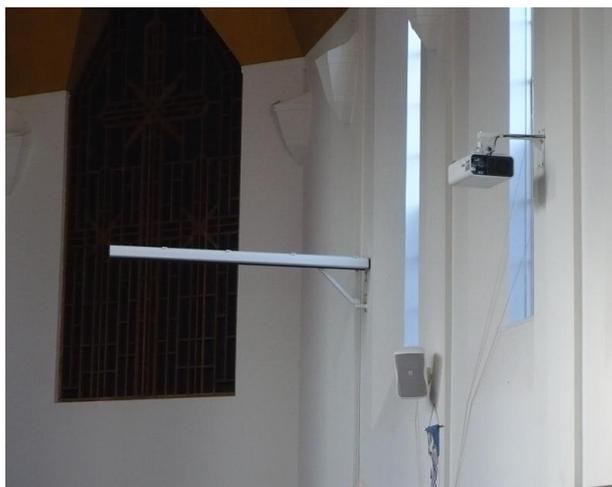
Sanyo 6500 lumen projector and custom screen that folds back discreetly against the wall when not in use
