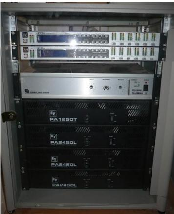
Main rack housing 6 channels of amplification for the ZX1is, 100v line amplifier for choir system and DC-One digital speaker processors
