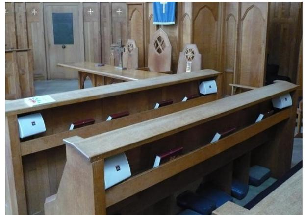
A compact monitoring system installed within the choir stalls provides clear and locally adjustable sound from a single volume control. Powered via 100v line technology allows further speakers to be added in the future.
