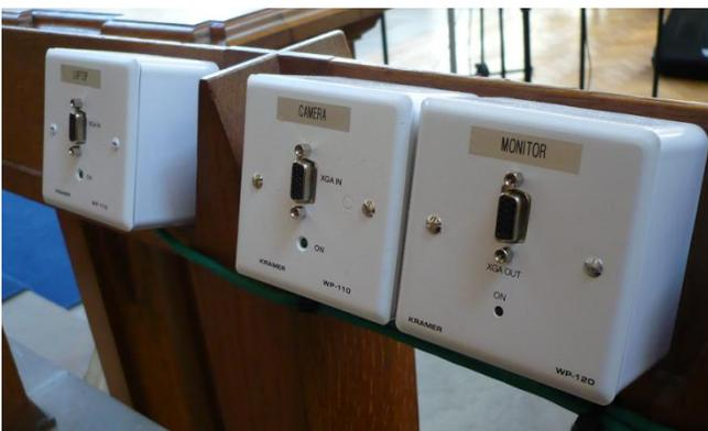
All visual connectivity utilises Kramer Twisted-pair (cat5e) distribution. Three active Kramer WP-110/120 plates on the platform are installed for laptop and roaming camera input with a monitor output for a TFT/LCD display.
