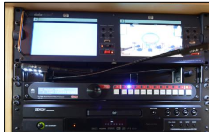
Part of the AV console rack showing a dual Datavideo preview monitor and TV-One Switching-Scaler
