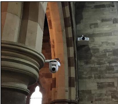
A Christie LW-751i 7,500 lumen projector for the main central screen and Sony SRG-300HW full HD motorised PTZ camera for projection, recording and online streaming.
