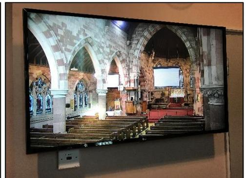
High definition camera images with audio is relayed to the crèche LED monitor. A local HDMI input allows the display to be utilised for independent meetings.
